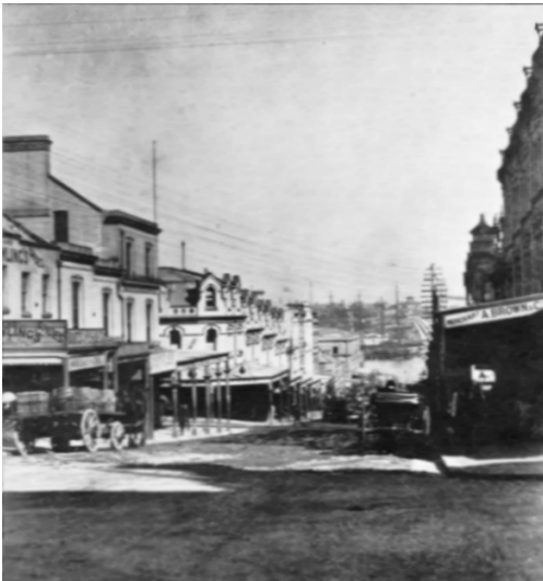
merchant traders, with some professional Erskine Street 1871 looking west to Darling Harbour – Evidently, street of long established tradesmen and people.
