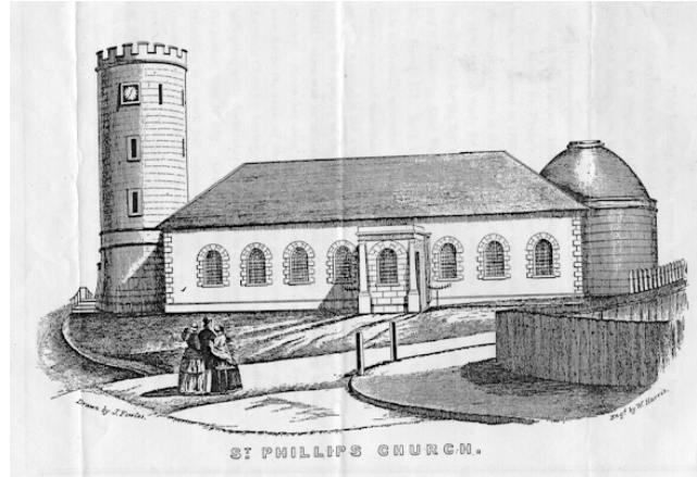
St Phillips. A square tower 150' high had been built in 1797 and used as an observatory and clock tower. The foundations for the church were begun in 1800 but it wasn't consecrated until 1810, although meetings were able to be held in it from 1808. It was replaced by the current building in 1856.
